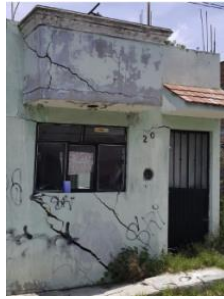
House fissuring and cracking (FIGUEROA-MIRANDA et al. 2018)
