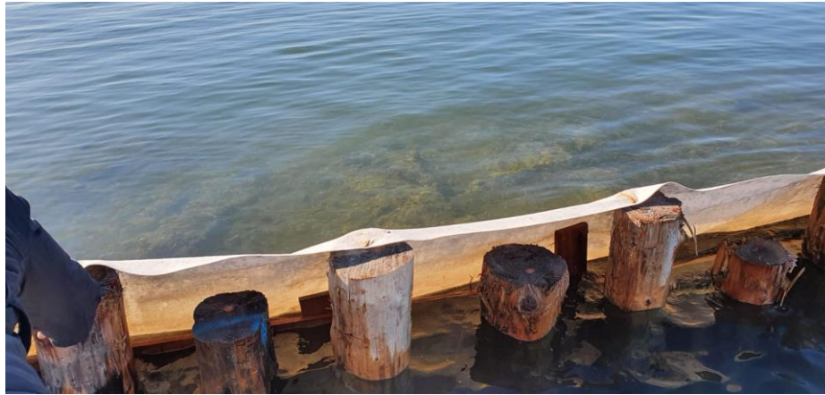
Sediment retention structure build during summer 2021
